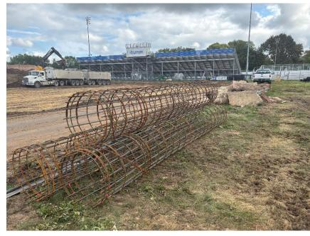
LCHS Steel reinforcement for foul pole foundations
