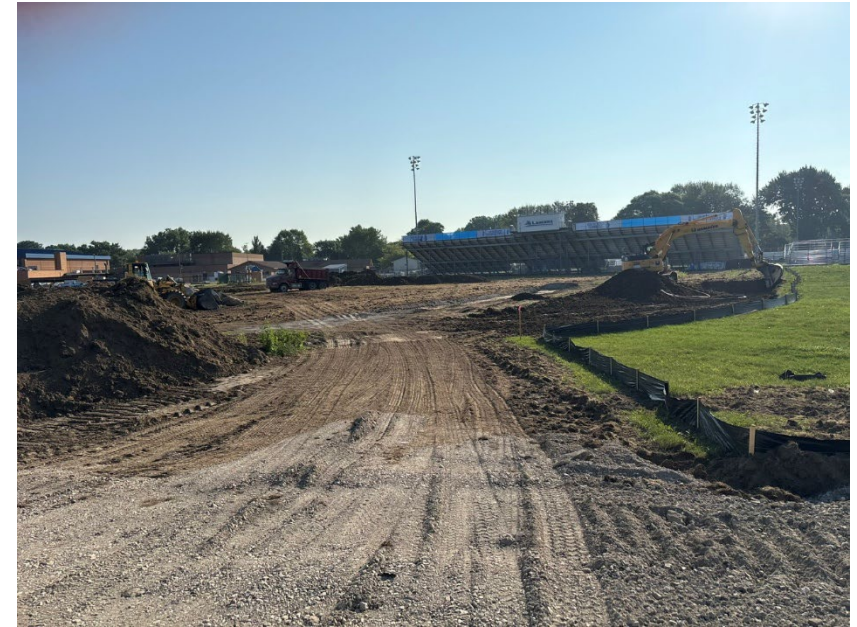
LCHS baseball field Topsoil Removal
