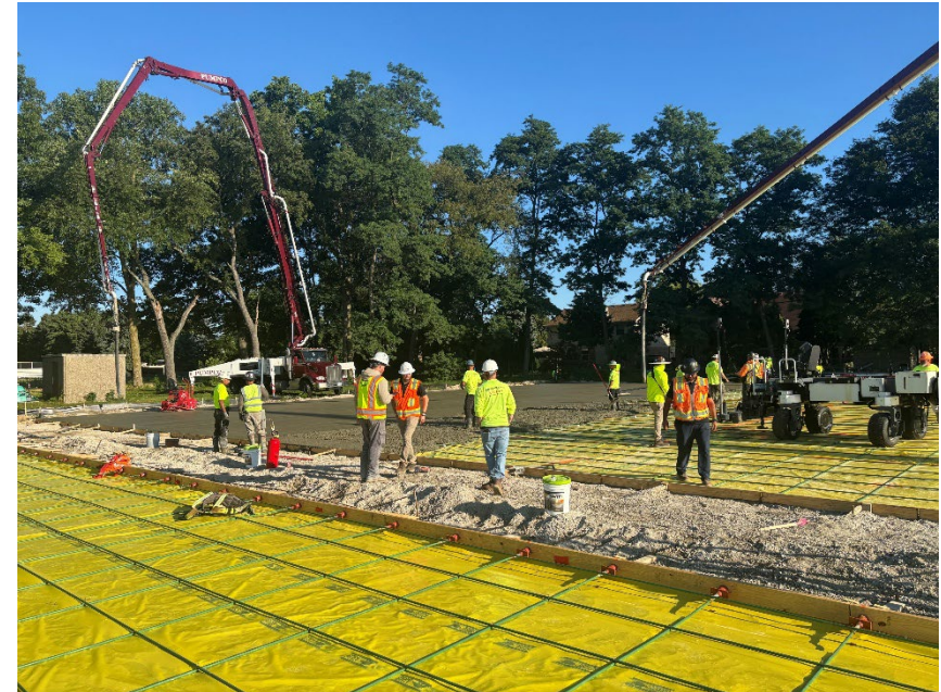
HSN placing tennis court concrete
